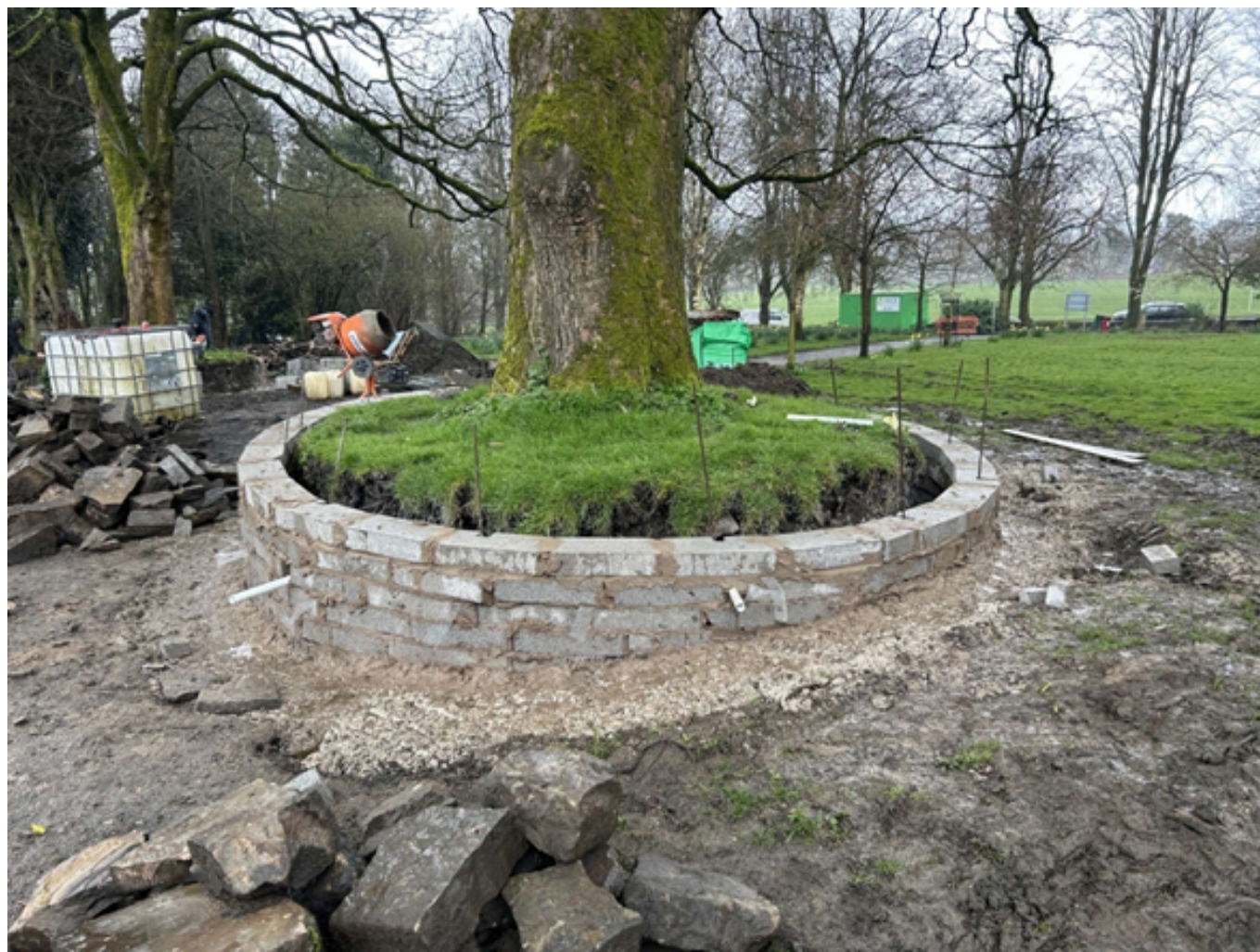
Building new tree walls, 4th April 2024
